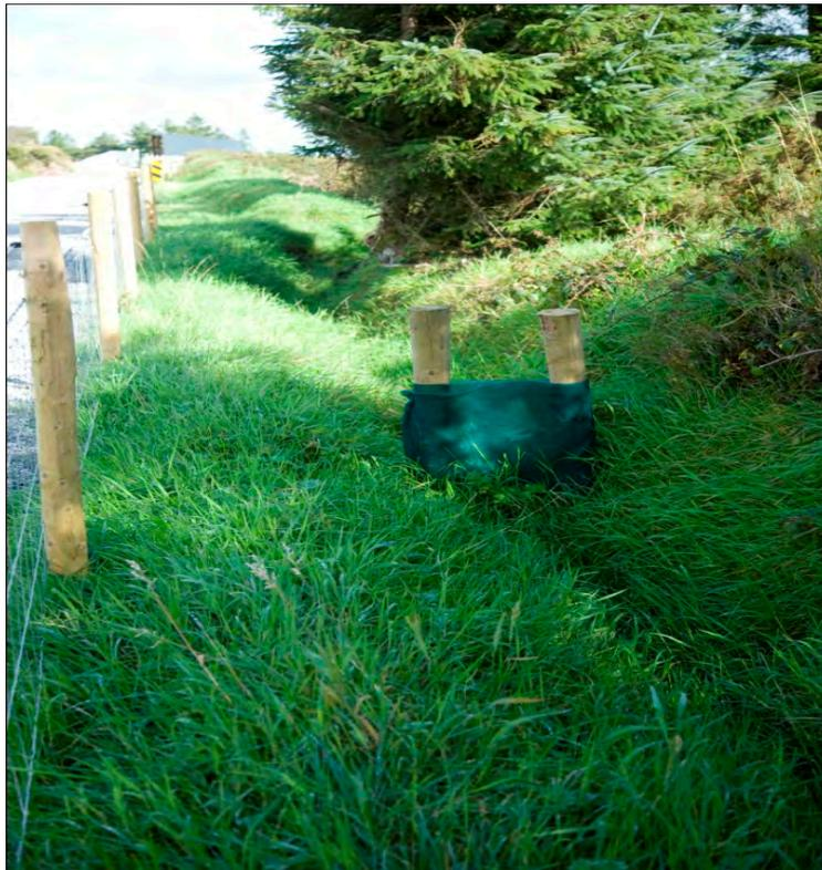
Figure 4-4: *Silt Trap across Grassed Swale*
