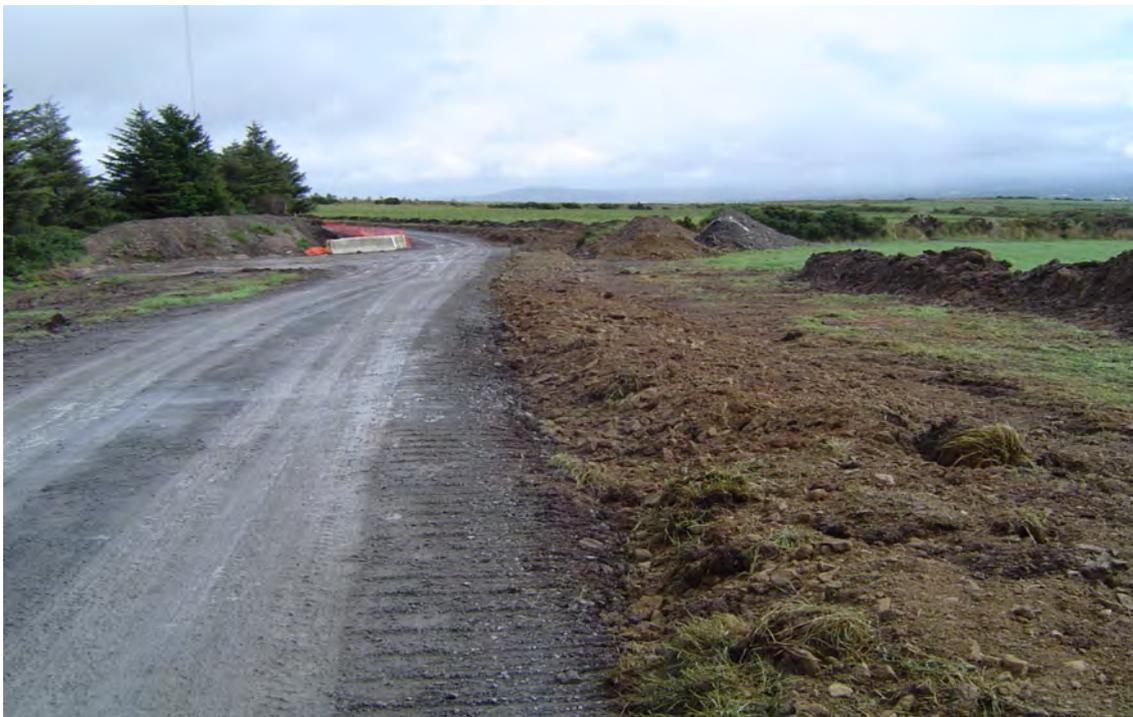
**Figure 4-7:** *Backfill over Cable Trench*
