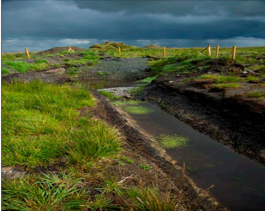
**Figure 4-2:** *Swale draining to Settlement pond*
